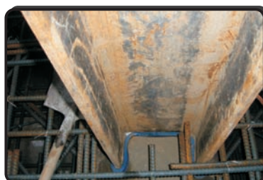
H型鋼皂土條防漏
