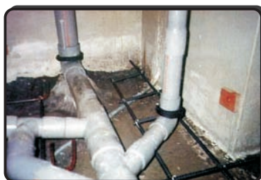
PVC管皂土條防漏
