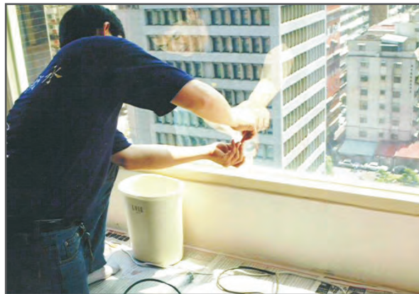
步驟二:橫料低壓灌注 step two: horizontal material low pressure injection
