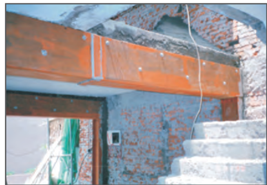
樑柱鋼板包覆灌漿補強 Pile steel board wrapped injection strengthening
