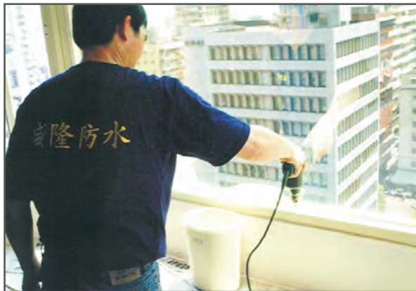
步驟一:鋁料鑽灌注孔 step one: aluminum material drill injection hole
