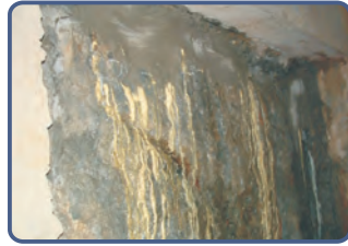
【先灌注止水】 stop leaking by injection first
