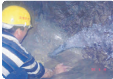
2.大速凝水泥急結凍水 Quick coagulating cement quick
