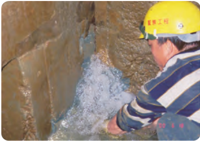
1.大底湧水現況 Plate water gushing
