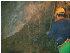
地下室連續包泥處理 Basement continuous earth covering disposal
