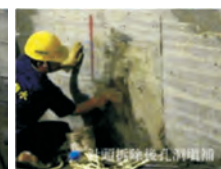
Fill cavities after demolishing pinheads
