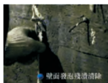
Clean off foaming leftovers on walls
