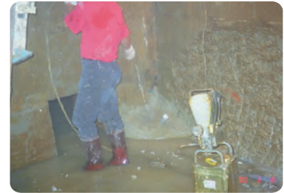
3.高壓灌注斷水 High-pressure injection and water supply cut off
