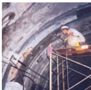
隧道止漏 Tunnel Leaking sealing
