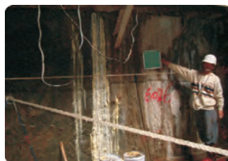
連續壁體止漏 Diaphragm wall leaking sealing
