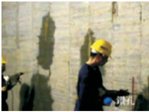
一、鑽孔 Holes drilling
