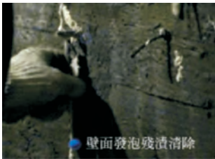
四、壁面發泡殘漬清除 Clean off foaming residuum on walls
