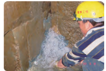
大底湧水止漏 Plate water gushing leaking sealing
