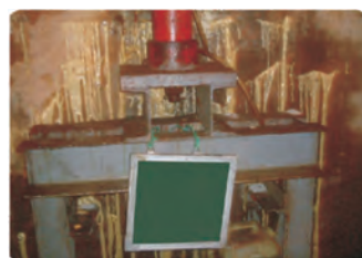
電梯機坑止漏 Elevator trench leaking sealing
