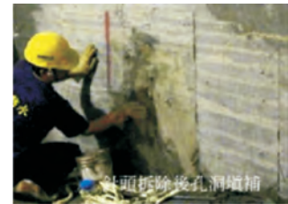
六、針頭拆除後孔洞填補 Fill cavities after demolishing pinheads
