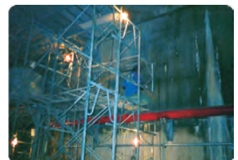
地鐵牆面止漏 Subway wall leaking sealing
