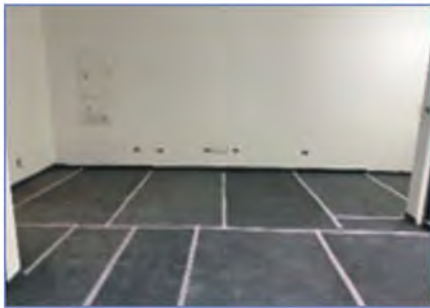
4.鋪設SL-570橡膠隔音墊
