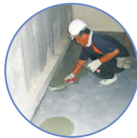
3.週邊地坪修補 Surrounding terrace repair
