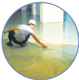
5.塗佈EPOXY中塗 EPOXY middle coating
