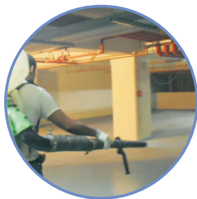
6.噴灑(石英砂+金剛砂) Spraying (silicon sand and carborundum)
