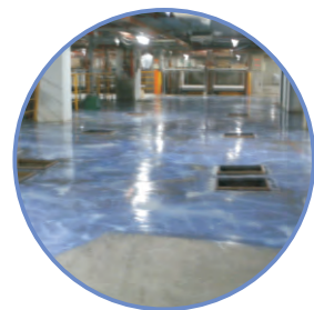
4.塗佈EPOXY底塗 EPOXY bottom coating
