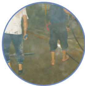
2.高壓清洗 High pressure washing
