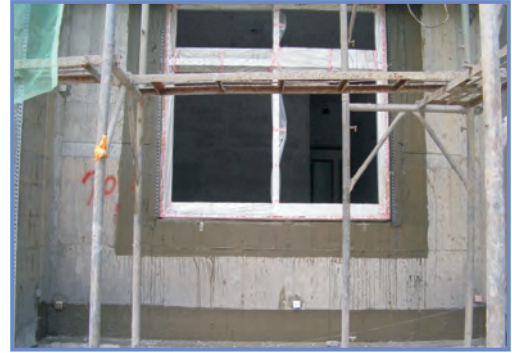
窗框.層縫防水 side of window hole waterproof
