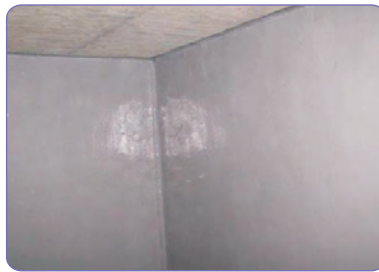
筏基坑 Foundation pit
