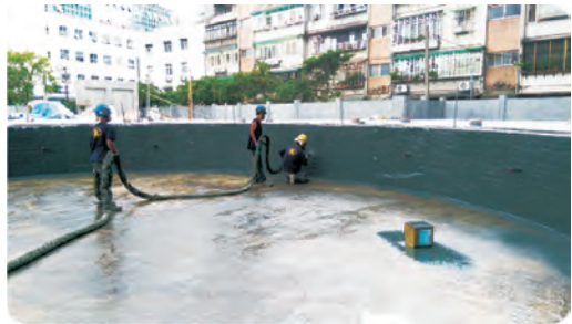
化學儲存槽防鏽蝕及保溫示意圖 Chemical storage tank(rust proof and thermal insulation)sketch map
